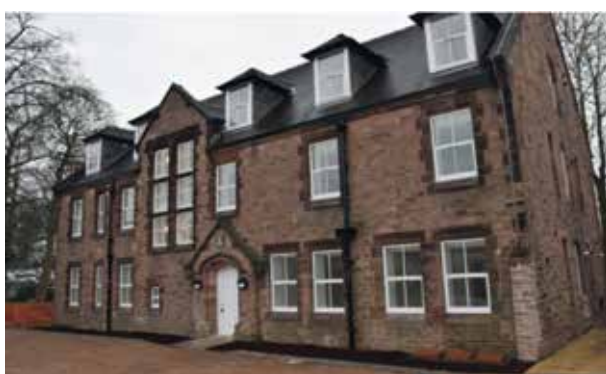
Henbury Building, Hope Park, Macclesfield – Purchased on 11 December 2015 for £2.8M
