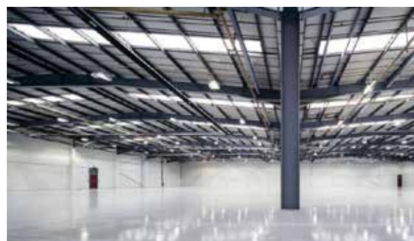
Refurbishments at Crawley, Woolborough Lane Unit D
